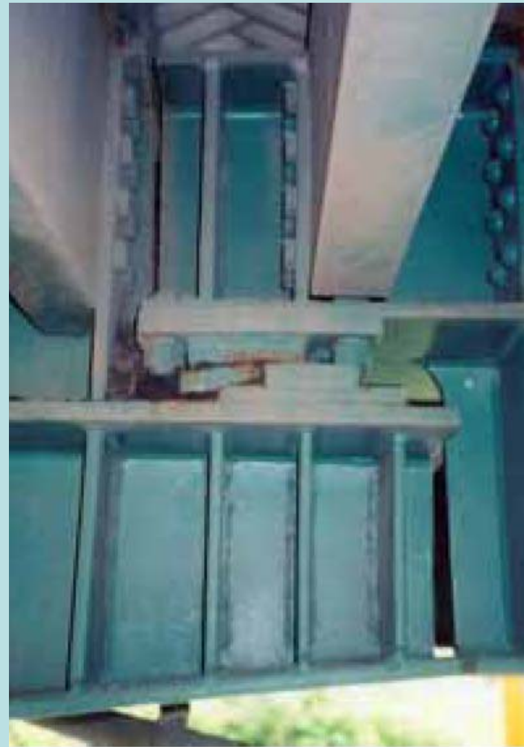
Sliding Plate @ Beam 5 NBL
