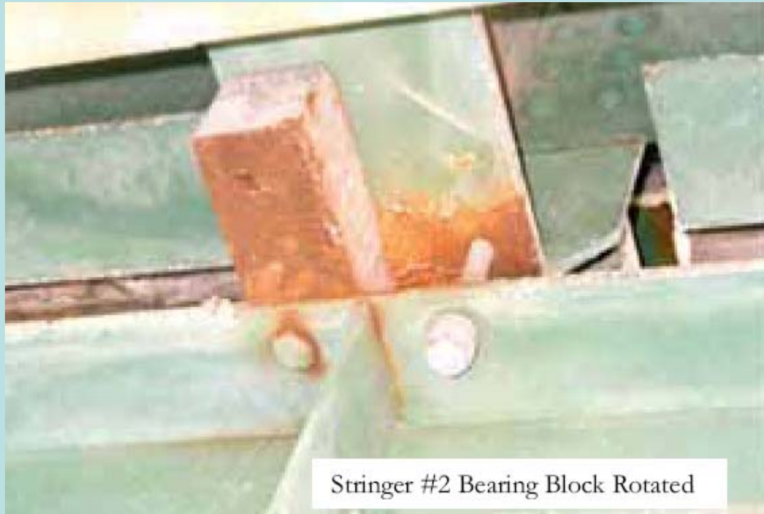
Stringer #2 (south side): bearing block has rotated 90°.
