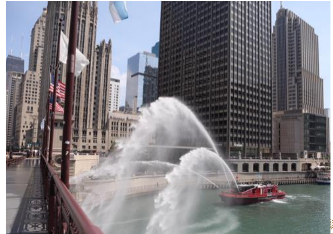
Joint closure during a heatwave in July 2018
