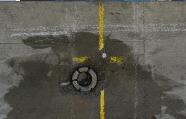
Exit of drillhead
