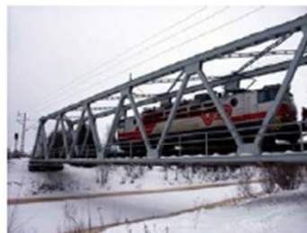
Steel beam bridges
