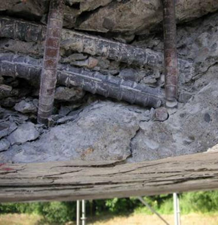
Stirrup rupture after yielding
