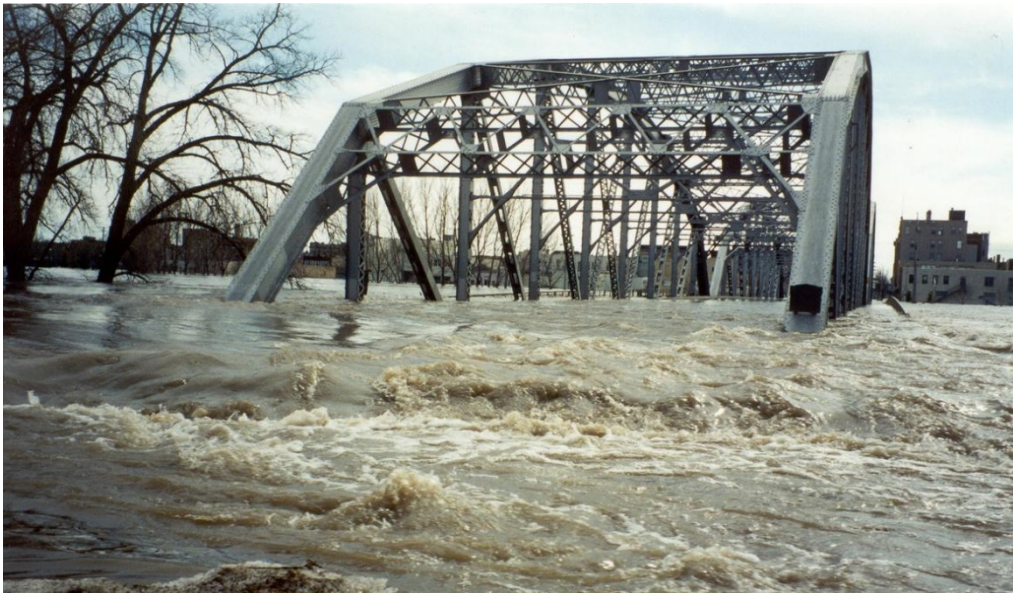
Flooding of the Sorlie bridge during the 1997 Red River of the North flood, Minnesota, U.S.A.
