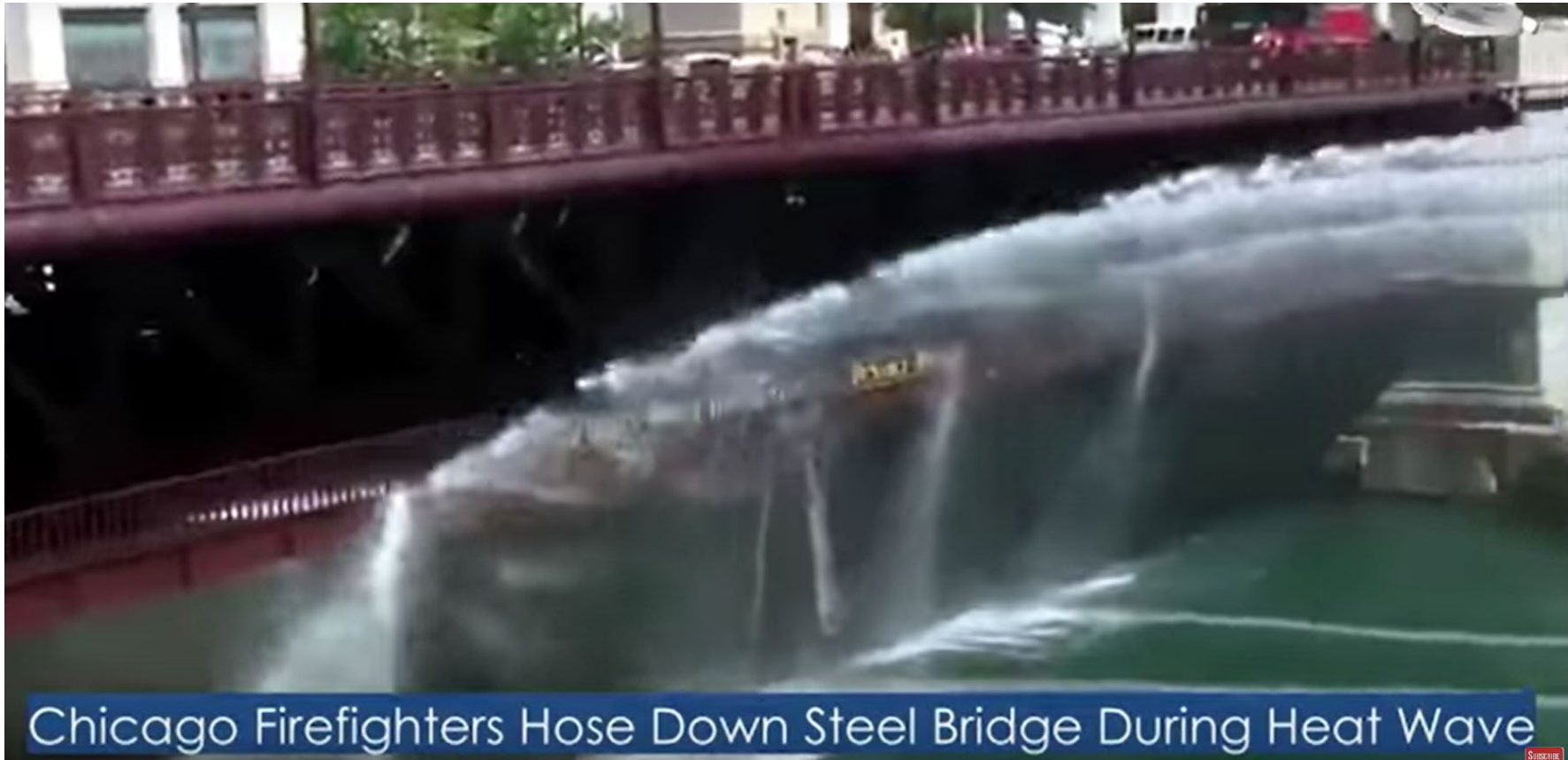
Joint closure of DuSable Bridge, Chicago, USA during a heatwave in July 2018
