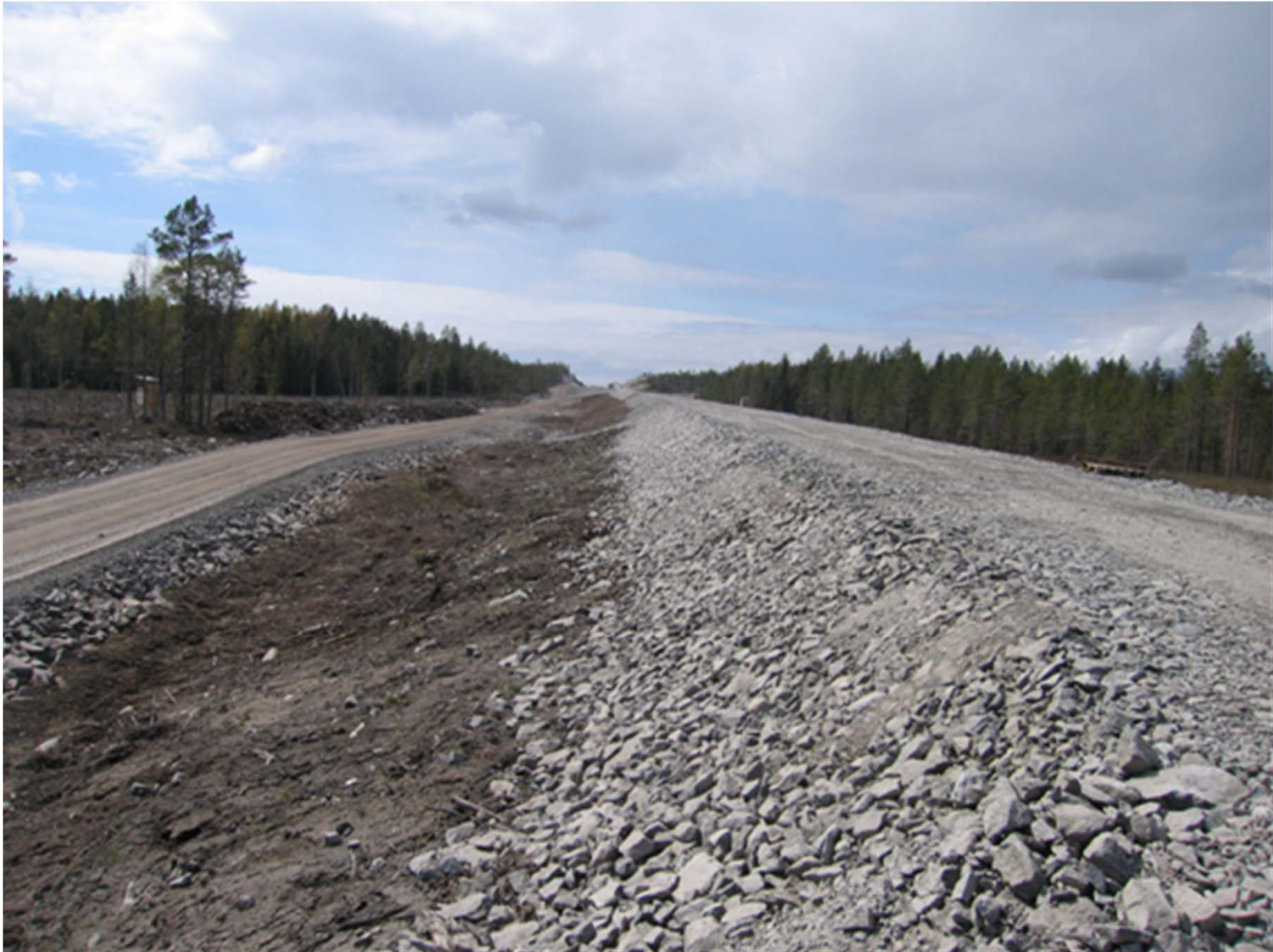
Railway track foundation. The service road is shown to the left.
